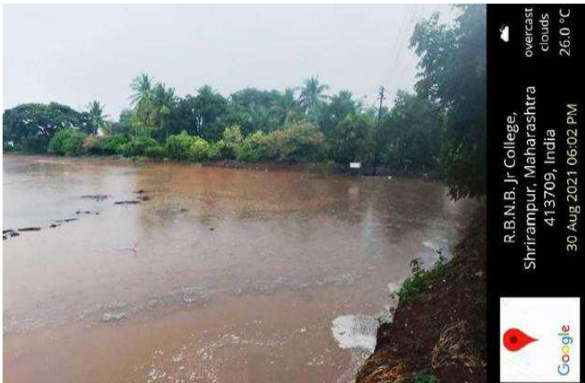
Construction of Bunds for rain water recharge
