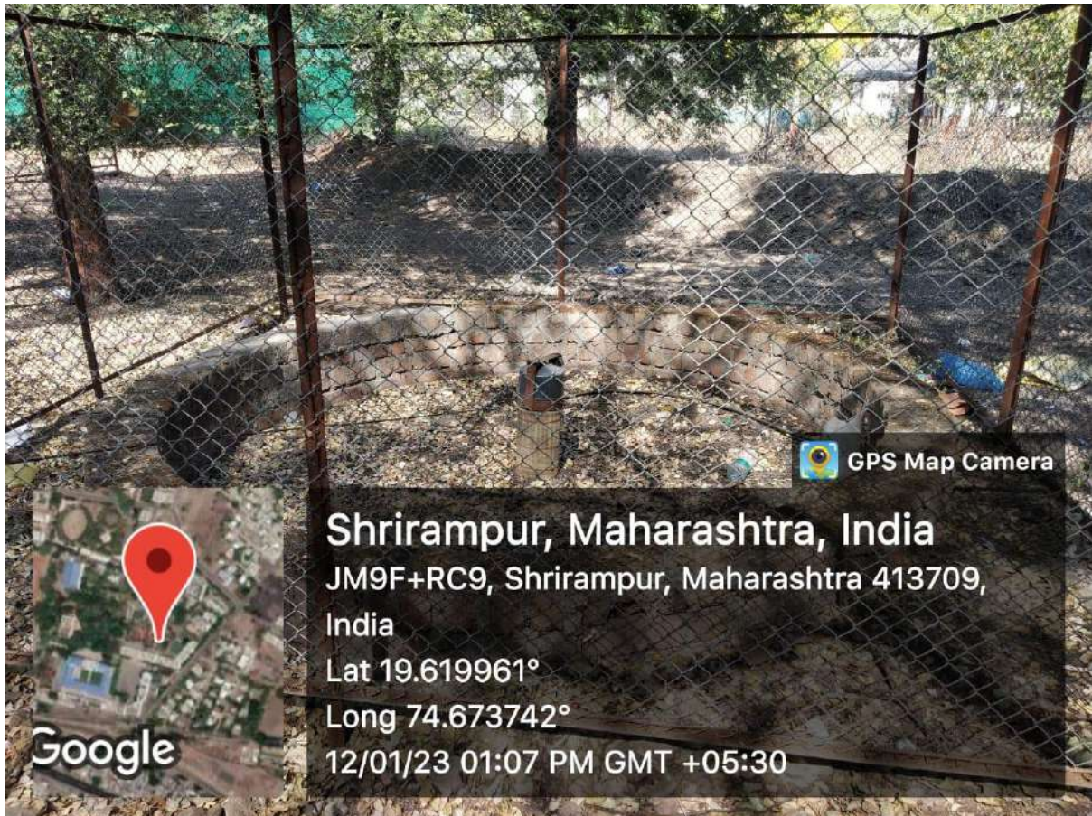
Bore well recharge Pit on College Campus
