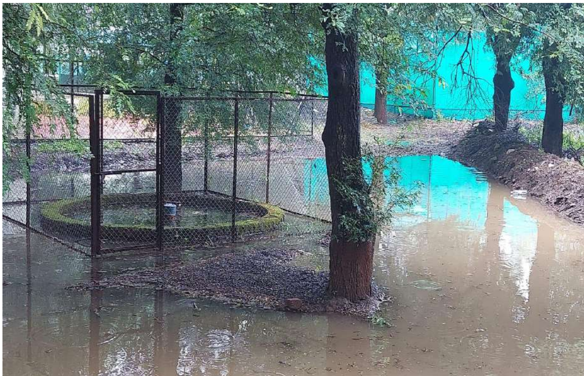
Bore well recharge unit near Wachan Katta
