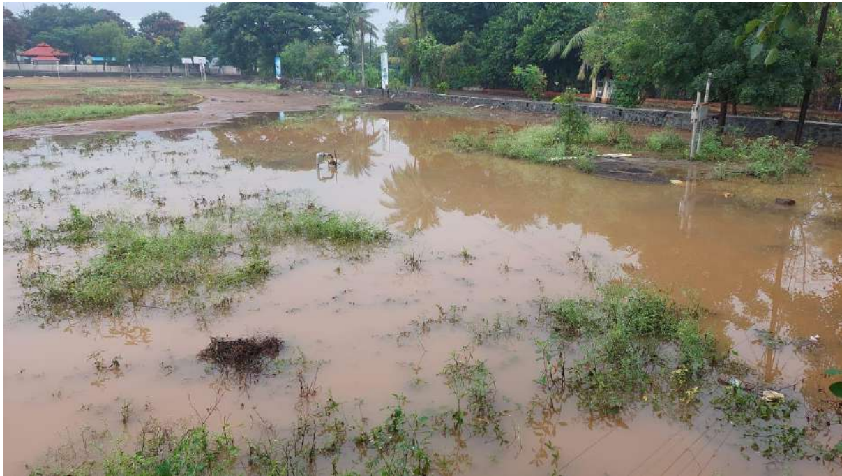
Construction of Bunds for rain water recharge
