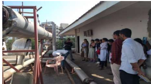
Visit to Parabolic Solar Concentrator
