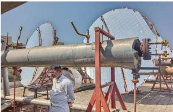
Parabolic Solar Concentrator
