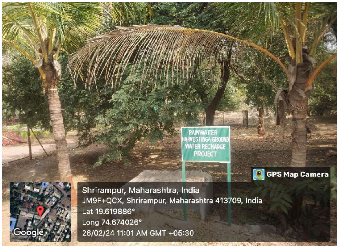
Roof-top rain water harvesting and ground water recharge in Tamarind Project
