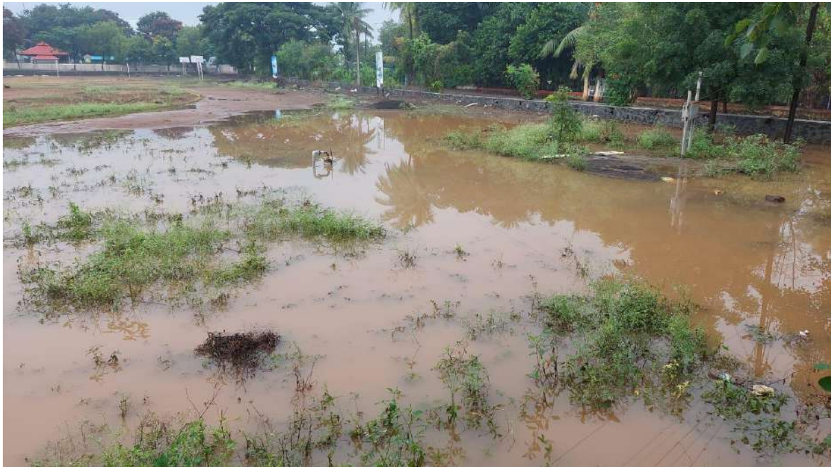
Construction of Bunds for rain water recharge
