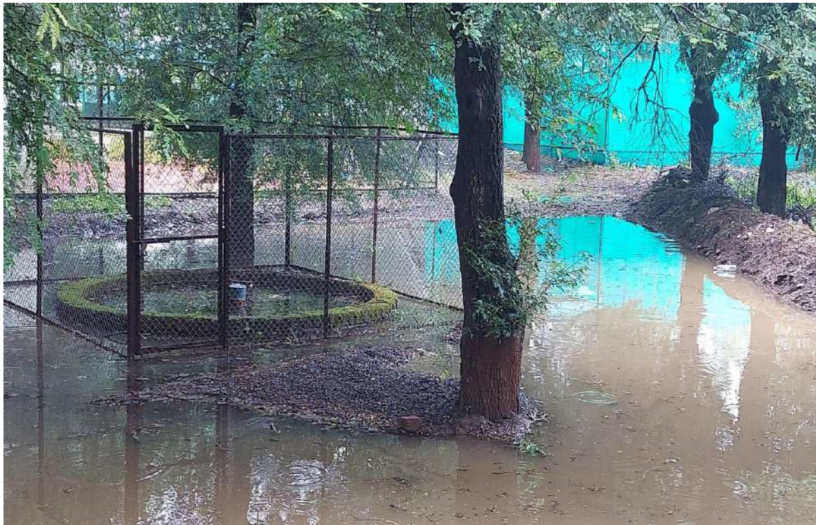
Bore well recharge unit near Wachan Katta
